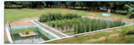
Constructed wetland for waste water treatment
